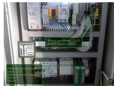
Fig. 17. Example of a screenshot of an AR system used to support diagnostic processes in an electrical panel (source: [27]).
